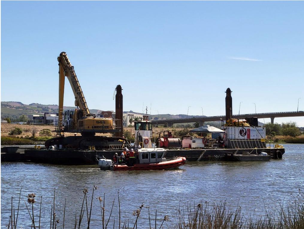
**Figure 5- An excavator dredge in operation on a river. Photo by USACE San Francisco District.**
